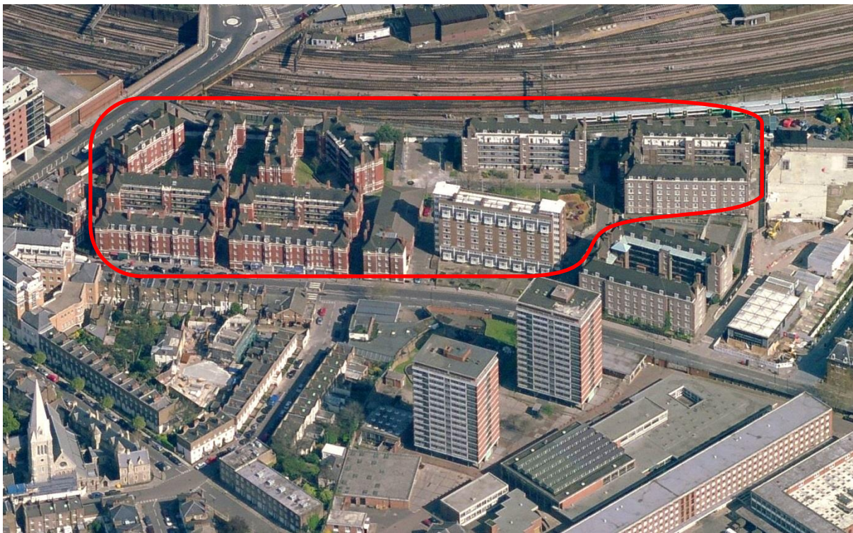
Figure 4 Aerial view of Ebury Bridge Estate
